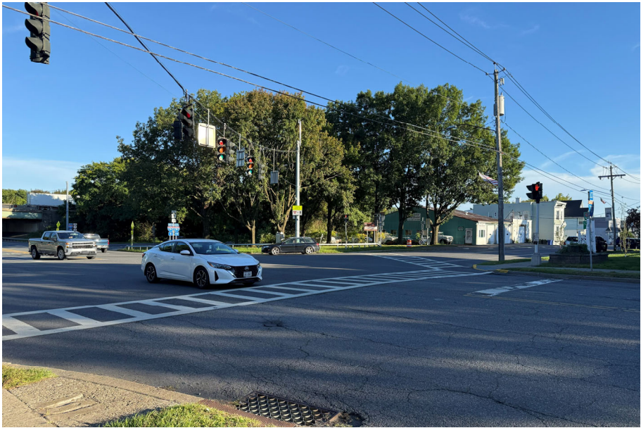
Above: Existing condition
